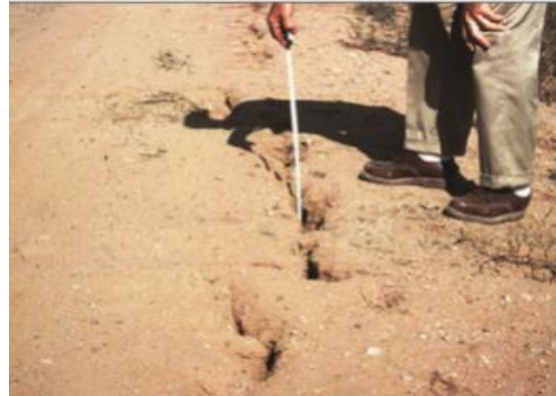
Longitudinal Cracks Indicate Dam Instability
