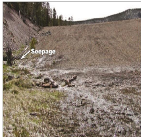
Abutment Seepage May Lead to a Dam Failure
