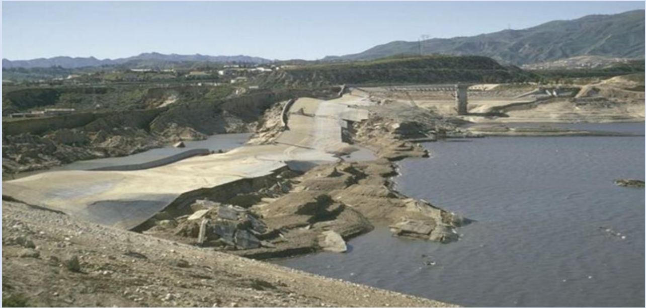
(Lower San Fernando Dam, California, USA after 1971 Earthquake – Failed due to Liquefaction)
